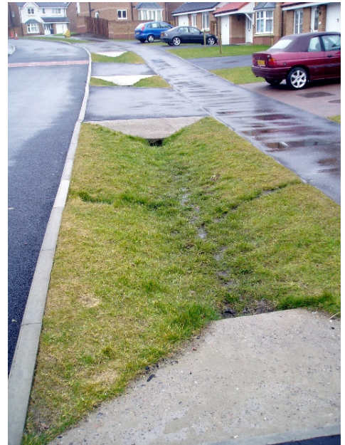
Figure 4-4. Photo of a swale. Credit: Susdrain .
