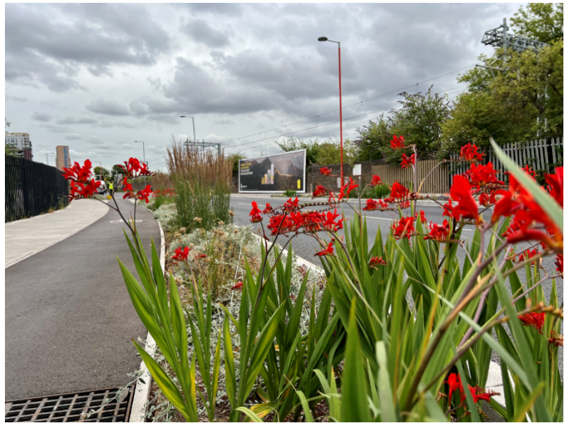
Figure 4-1. Photo of a rain garden. Credit: Meristem Design .
